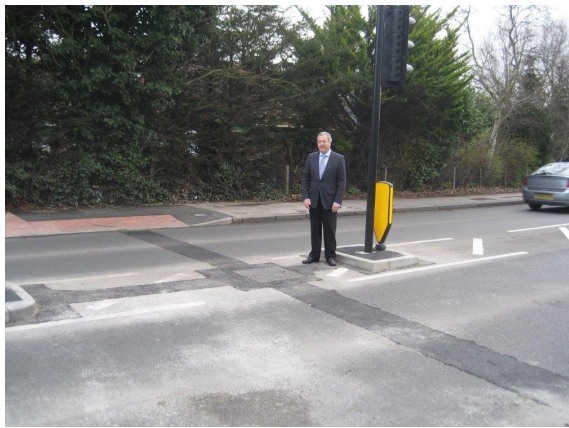
Checking the nearly finished toucan crossing in Gaston Bridge Road.
