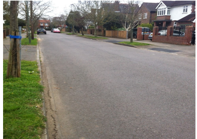
Ash Road Shepperton Green resurfaced
